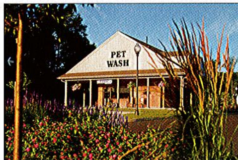
Cloister's three bay, self-service pet wash.
